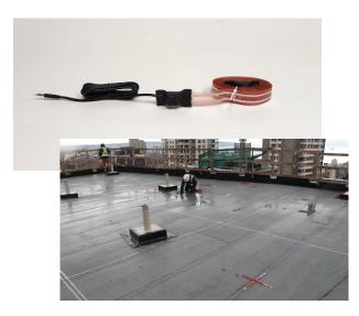
Moisture Detection Sensor (MDS) Tape is used for the detection of physical moisture within an assembly
