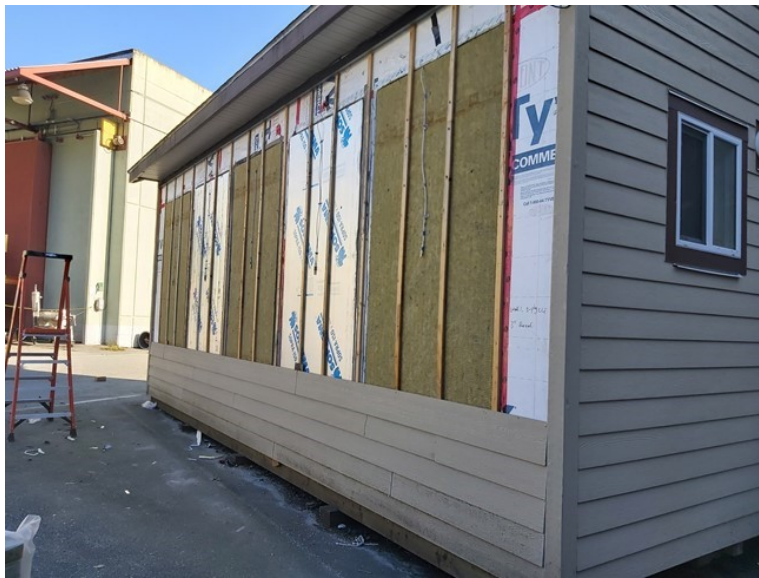
Figure 20. The exterior surface kept flush for installing continuous strapping and siding.
