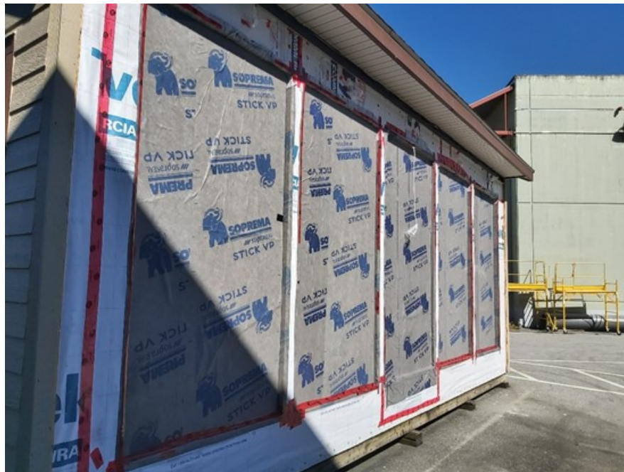
Figure 18. All test wall panels installed at the test hut.
