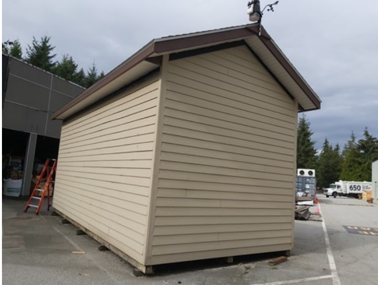
Figure 21. The exterior completed.
