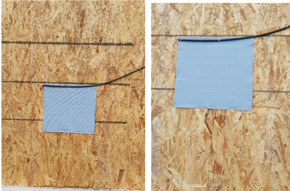
Figure 17. A new wetting pad fed with a water tube installed on the exterior surface of the OSB sheathing of wall 3 (left: S3; right: N3).
