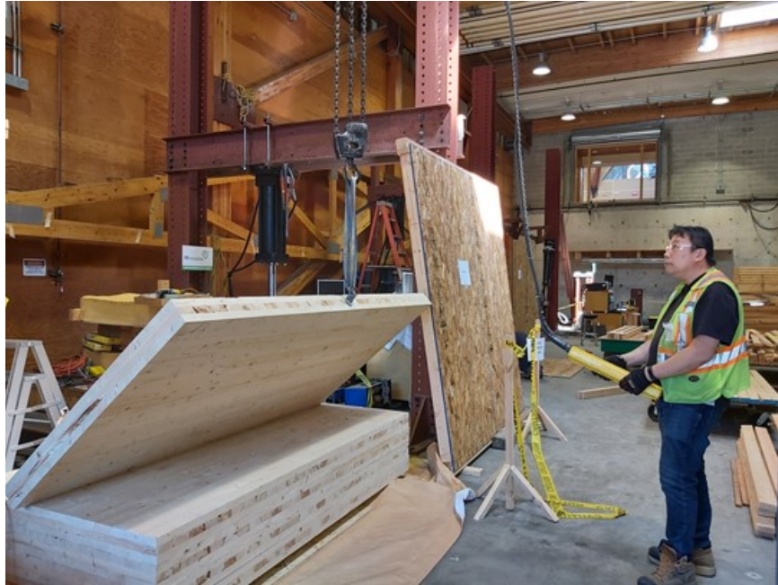
Figure 13. CLT panel being lifted for pre-preparation.
