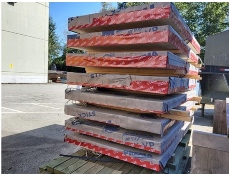
Figure 16. Piles of pre-prepared CLT panels prior to site installation.
